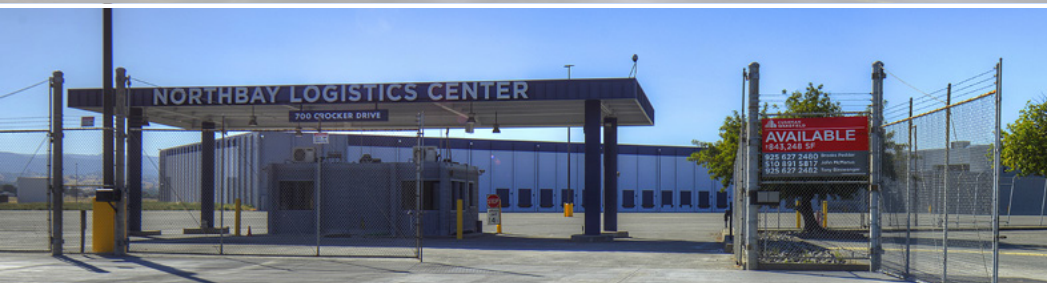
GUARD SHACK & SECURE ACCESS
