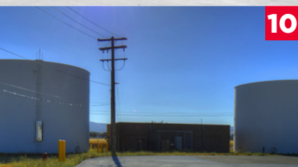
Water Tanks and Sprinkler Pumps
